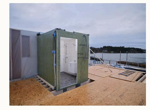
In this configuration, the bathroom doesn't just house plumbing fixtures - it becomes the technical backbone of the apartment, where water, heating, ventilation, controls, and safety sensors converge into one coordinated module.
